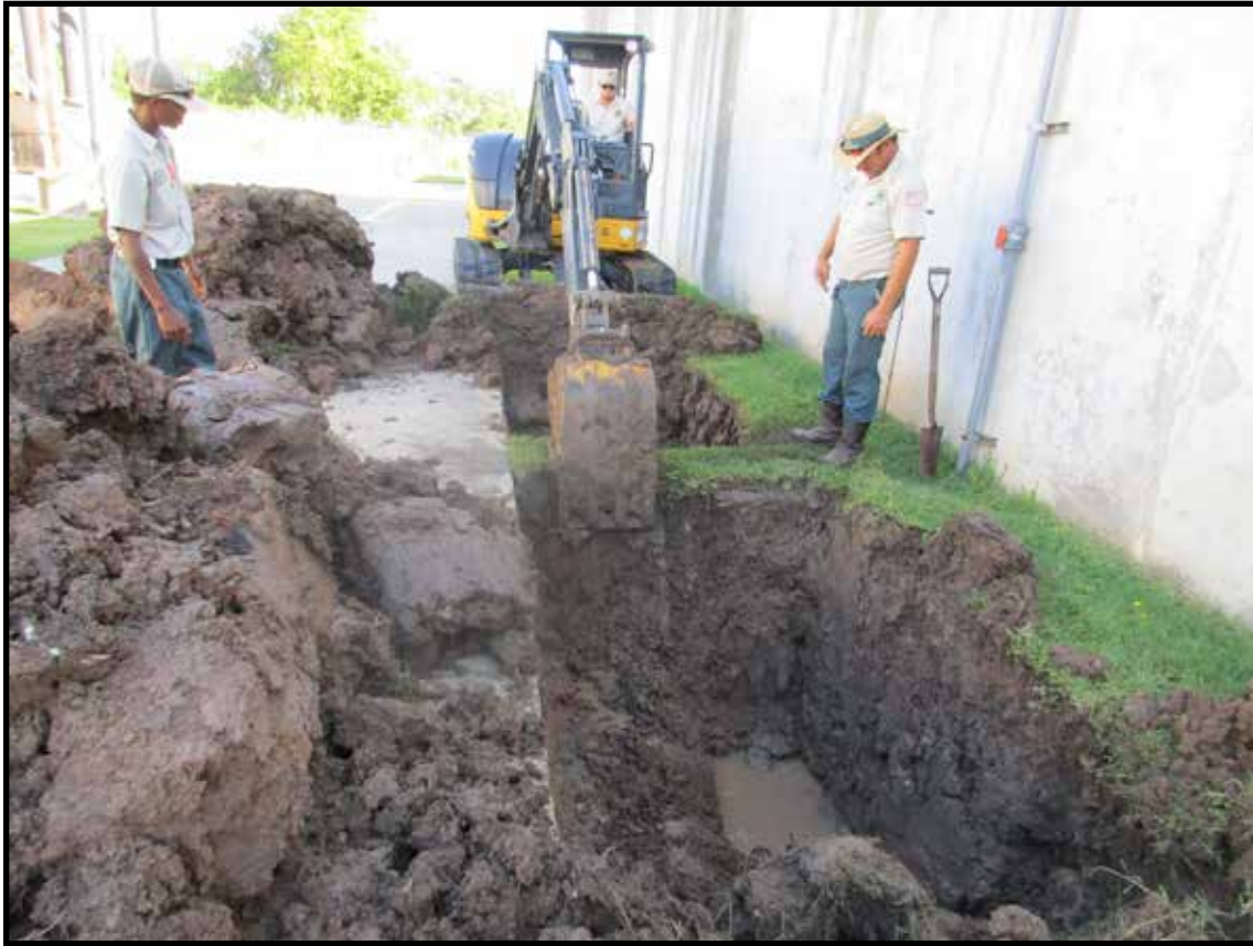
Utility Crews Repairing a Pipe Leak
