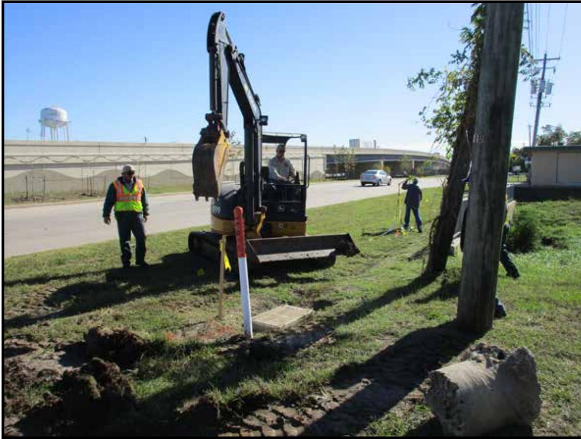
Utility Crews Working Near Lift Station #1
