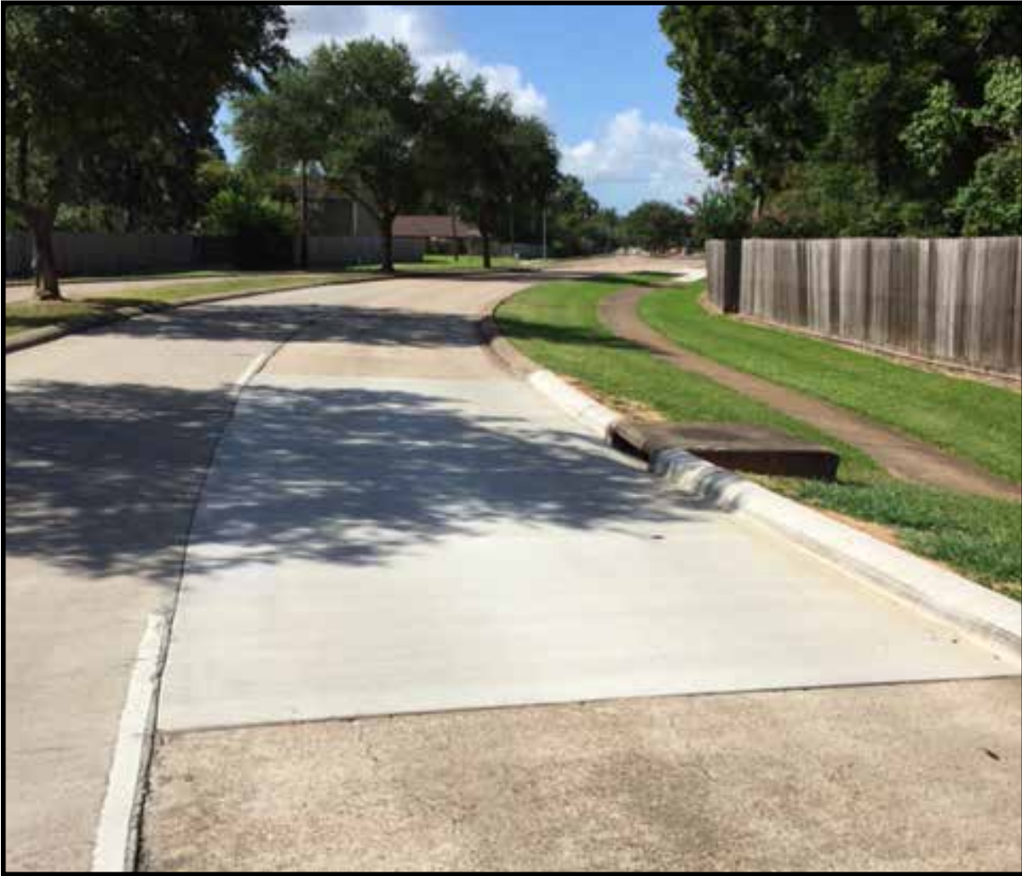
Newly Finished Street Panel Replacement on Yaupon Drive
