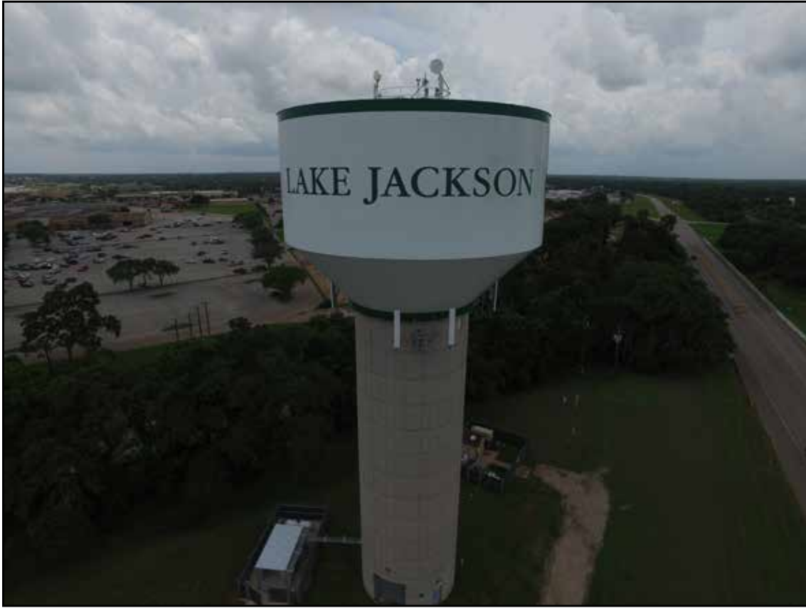
Lake Jackson Water Tower at Dunbar Park
