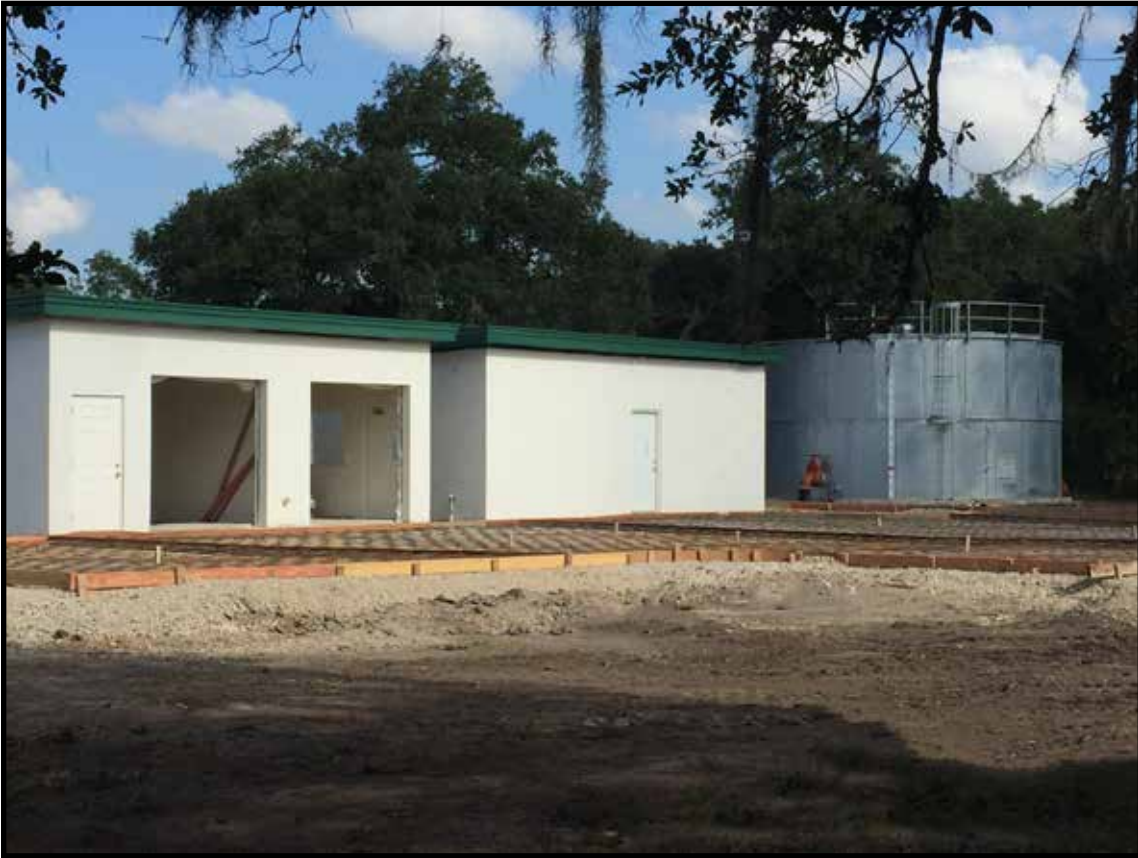
Construction of the North Water Plan Near the Airport
